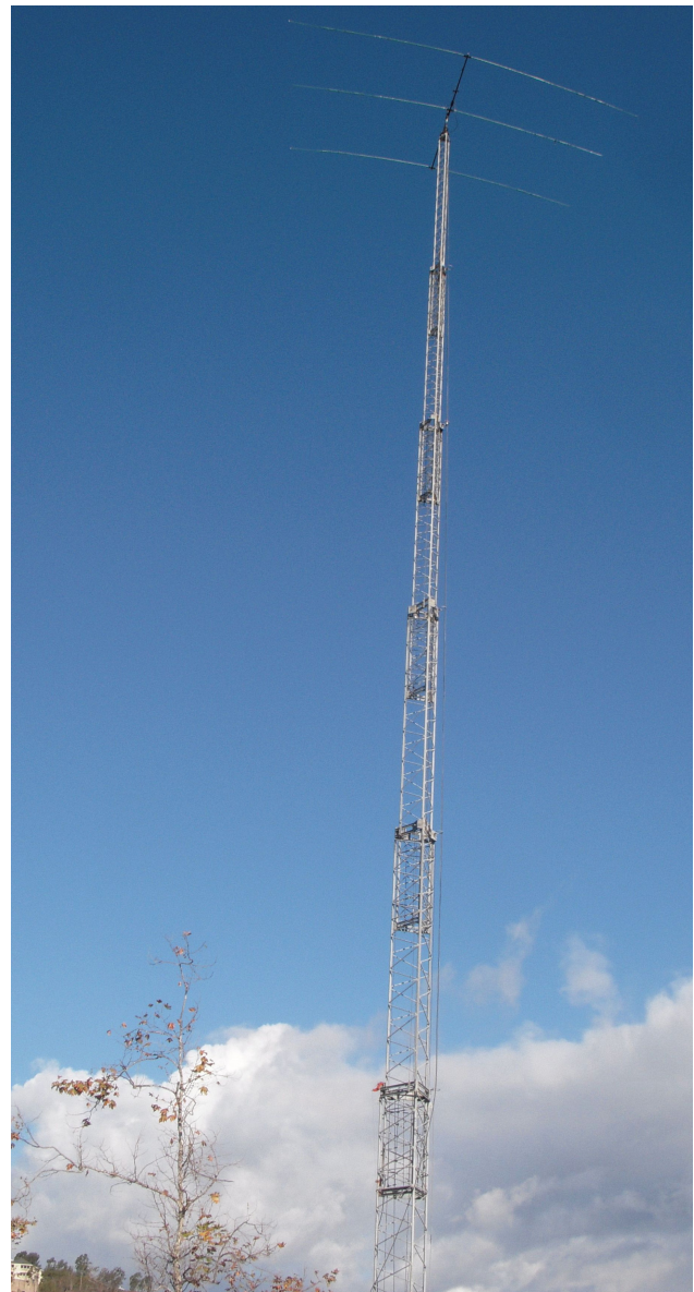
Ham events need antennas. The El Cajon Amateur Radio Club tower.
