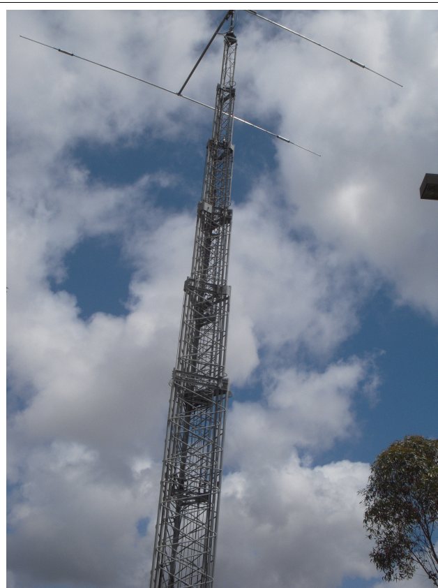
Not all portable ham towers are small. This one is only cranked up part way.
